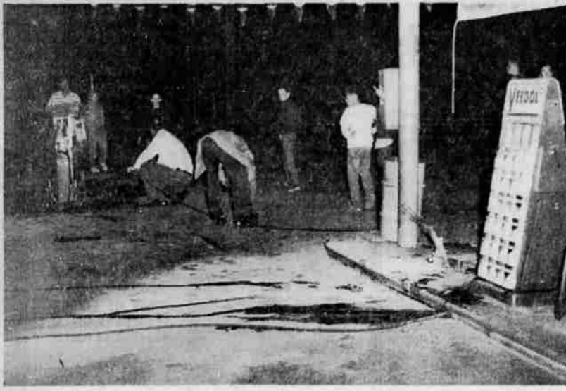
GASOLINE FIRE —A motorist drove away from a gasoline pump at Tidewater Oil company, Oak Grove rd. and Jacksonville highway, Tuesday before the filler hose was removed from the gas tank. The resulting jolt, which pulled the pumping unit from its stand, caused a wire shortage, and the gasoline in the hose caught fire. Medford firemen contained the fire in the hose and pump, but some damage to the pump was noted. (Knackstedt photo)
