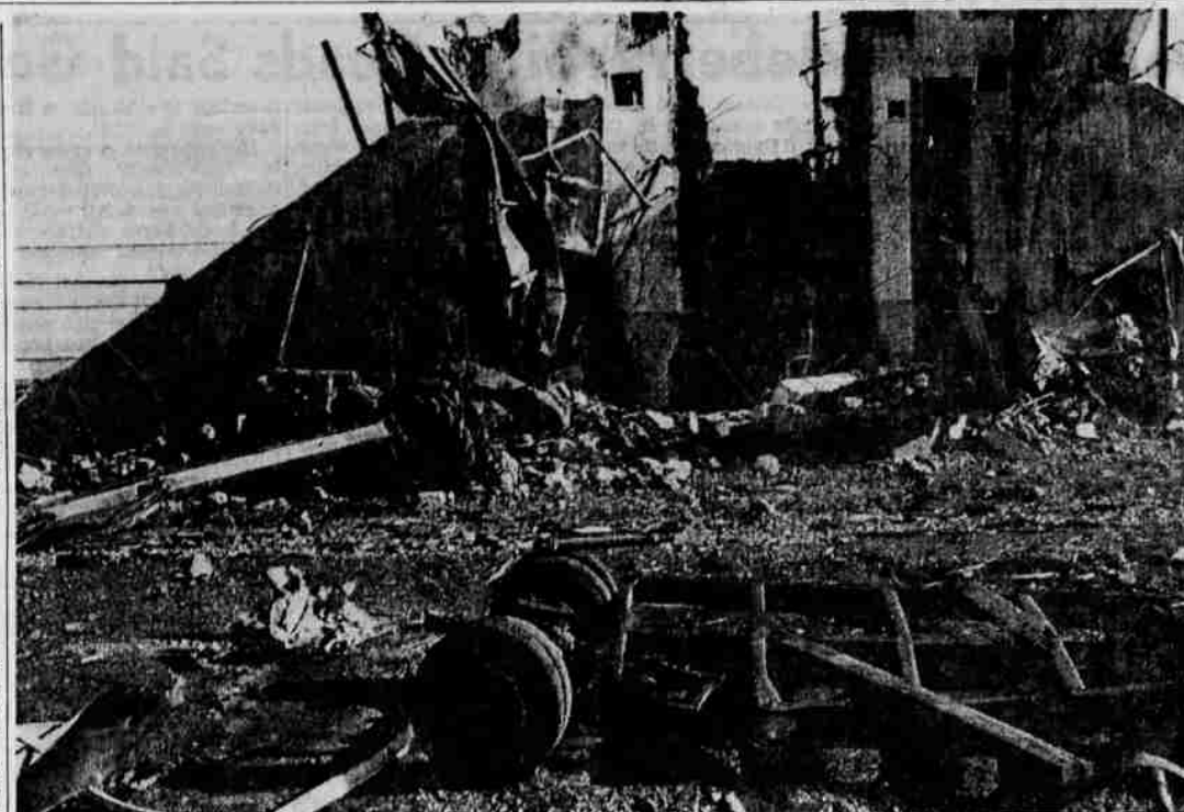
BUILDING DEMOLISHED —This was a solid fuel curing building at the Hercules Powder Company in Bacchus, Utah, before it was demolished by an explosion Thursday. The violent blast left three men missing and presumed dead and three injured. (UPI)
