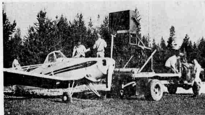
SECOND PHASE—Operation aerial fish lift in second phase of transferring fingerling trout from aerated hopper aboard a flat-bed truck into the aerated hoppers aboard the aircraft. (Game Commission photo)
