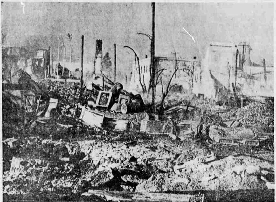
EXPLOSION CRATER —The above picture, made Aug. 7, 1959, shows a portion of the devastation in Roseburg after an explosive-laden truck exploded in the downtown area. The picture was made at the edge of the crater where the truck had stood. (UPI)
