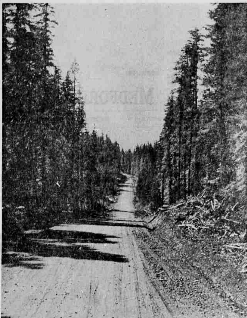
ACCESS ROAD —The bureau of land management's Keno Access road, shown here, was accepted as completed during the past three months. The 27-mile road will tap
