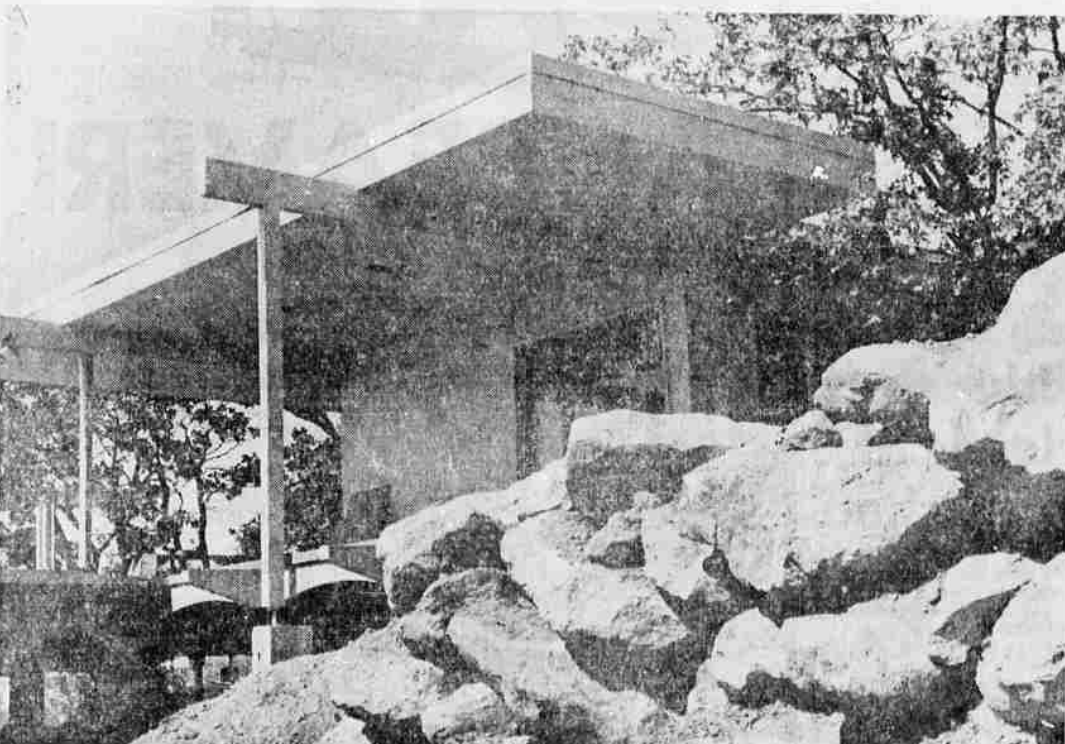
Built to fit into a hill on the east side of the valley, the new E. H. Loveness home is provided with decking most of the way around the house for the convenience of outside loungers. Alexander Diepenbrock designed the house around the trees and natural boulders to form a shady setting. This view of one portion of the structure shows the manner in which it is constructed on the hill.
