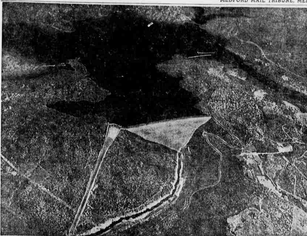
VIEW OF DAM —This is an artist's view of the Oroville dam and spillway on the Feather river in California. The dam will rise 735 feet from the river bottom and will be the highest dam in the United States. It will be the key to California's multi-billion dollar water development program. (UPI)
