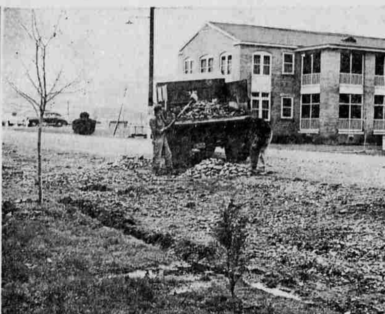
CLEANING GROUNDS —This is the way Camp White looked when work started on the Domiciliary back in 1950—covered with stones and bare of trees. Culverts have replaced ditches and all buildings have been repainted and reroofed.
