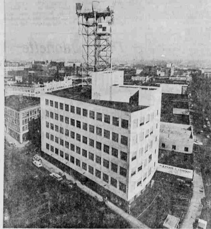
SWITCHING CENTER—Medford direct distance dialed calls will be channeled through the sectional switching center located in this building in Portland.
