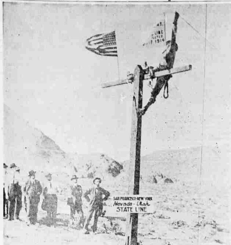
BEDECKED WITH FLAGS—Last pole on the first transcontinental telephone line near Wendover, Utah, was bedecked with flags and signs for the meeting of wires linking the East and West in 1914.
