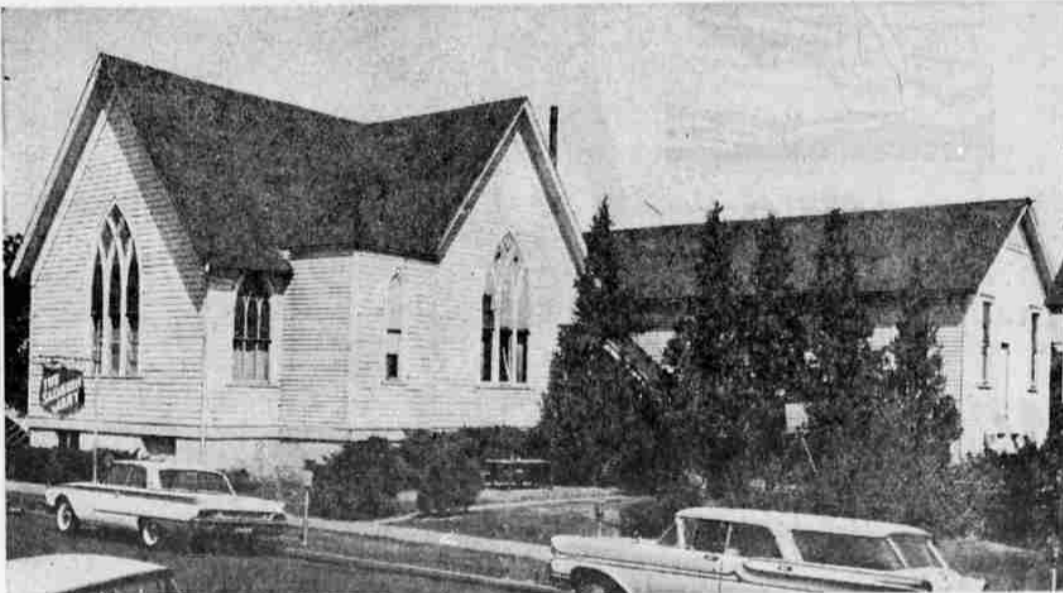
The Army's former headquarters and Community Center at Fourth and Bartlett sts. was condemned last February by the city because it was "unsafe for occupancy." The building, originally a Methodist church built in 1890, was purchased by the Medford Corps of the Salvation Army in the early 1930's and has been used by them ever since. (Salvation Army Photo)
