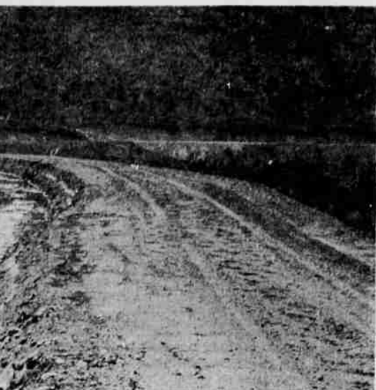
from Ashland to the Dark Hollow area. Beside the ditch is a dirt road wide enough so Talent Irrigation district trucks can drive along side the entire length of the canal.
