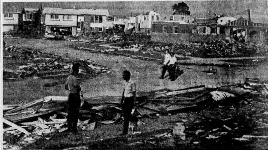
HOMES DAMAGED—A tornado raked a subdivision of new homes in suburban Oak Forest near Chicago, Ill., damaging 50 homes and injuring two persons. The twister, described as a "baby tornado" by the weather bureau, struck without warning. Residents of the area are shown walking through debris-covered streets. The twister was part of a storm front which brought thunderstorms, flash floods and lightning from the Rocky Mountains to the Atlantic Coast. (UPI)
