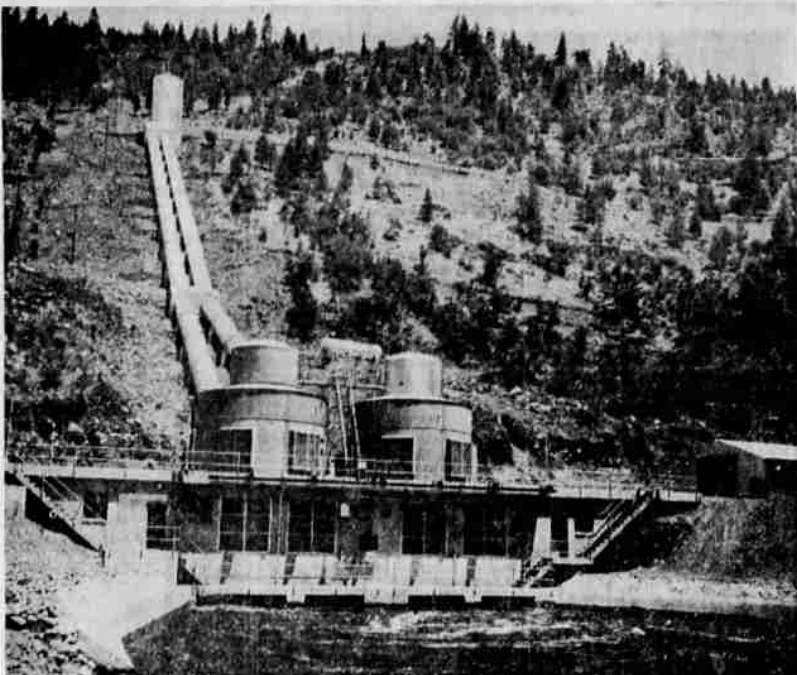
LARGEST IN DIVISION—Due to bear the name John C. Boyle Hydroelectric Project beginning Monday is this largest of Pacific and Light company's hydroelectric developments in the Copco division. Its two big generators can pour out 88,000 kilowatts of electricity at maximum capability. It is the first of seven planned for the Klamath river to harness its water resources for power and other beneficial uses.
