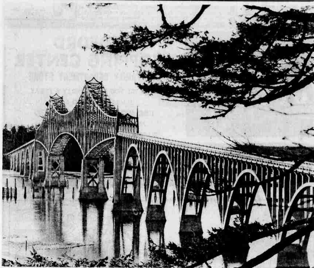
The McCullough bridge across Coos Bay, which is more than a mile long, is the longest of a series of bridges on the Oregon coast.
