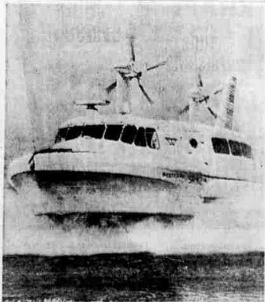
TRAVELS ON AIR—The SRN2 Hovercraft seems almost ghostlike as it is demonstrated on the Solent, the channel between southern England and the Isle of Wight. The craft, which rides on a cushion of air one foot over the water, reaches speeds of 70 miles an hour with its four jet turbine engines. It is designed to carry 75 passengers. (UPI)
