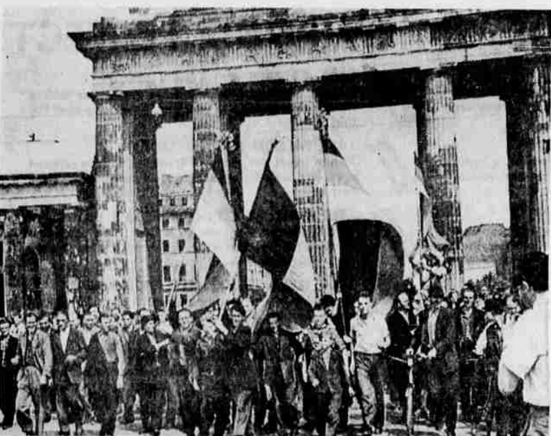
MARCH THROUGH GATE —Flag-waving East Berlin workers march through the Brandenburg Gate into the Western sector of the city after the start of the short-
