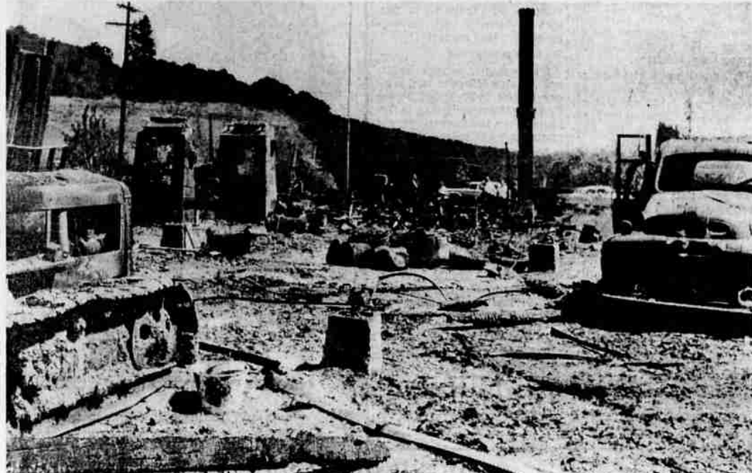
LANDMARK DESTROYED—This was all that was left of Stage Coach Orchards' packing house after Friday night's fire. Damage was estimated at $180,000.
