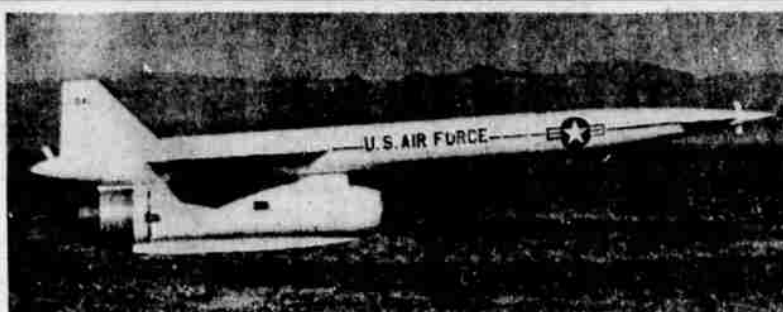
HOUND DOG IN FLIGHT — An Air Force XGAM-77A Hound Dog air-to-surface missile is shown flying over the White Sands Missile Range in this picture released by the Pentagon. The Hound Dog, produced for the Strategic Air Command by North American Aviation's space and information services division, has the capability for both high and low level flight following its launch from a B52 bomber. (UPI)
