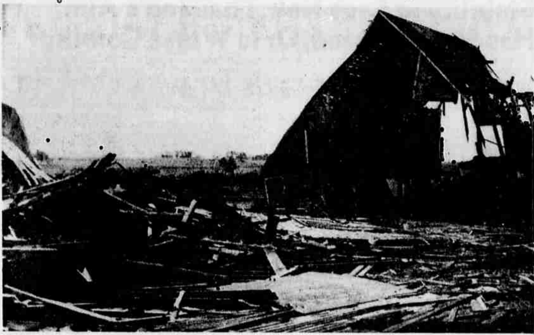
FARM BUILDINGS WRECKED - The Wilber Crandon farm buildings looked like this after a tornado cut a one-mile swath west of Gilman, Iowa. These two barns, a garage, the family car and their home were destroyed by the twister. Five members of the Crandon family were treated for cuts and bruises at a hospital. (UPI)
