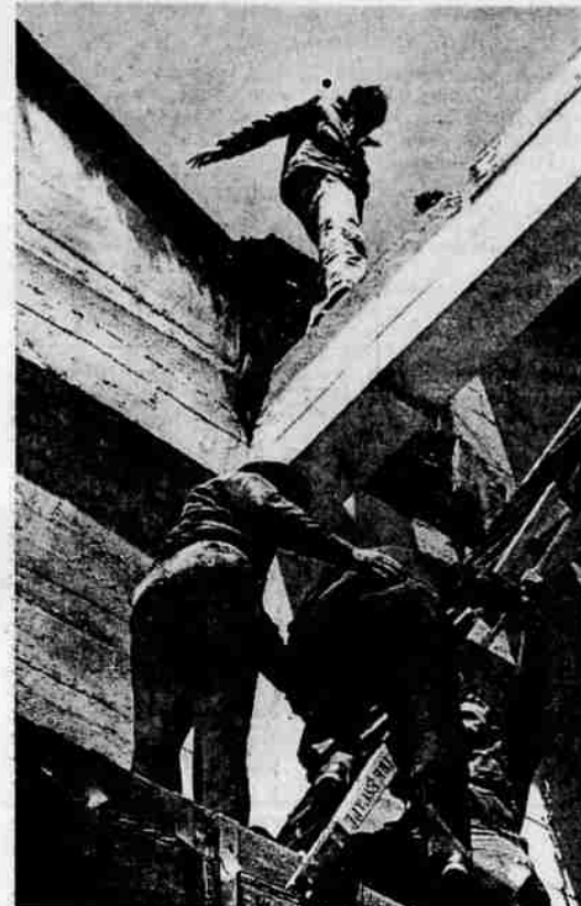
ARTIST RESCUED - Firemen go to the rescue of bearded, shoeless artist Heinz Dressler, top, on a beam atop the hull of a demolished warehouse in San Francisco. Firemen rushed to the scene when it was feared Dressler was attempting suicide. He was sunning himself, he told police, and was sorry he caused such a commotion. He also admitted he didn't know how to get down, so it's a good thing the firemen decided to investigate. (UPI)
