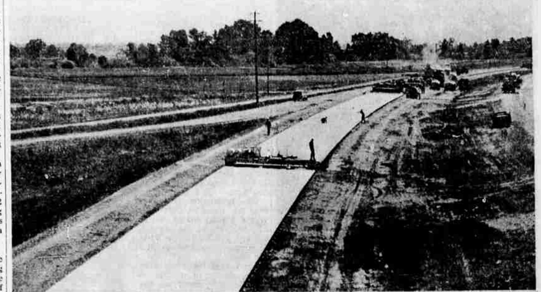
PAVING STARTED—Paving of the section of Interstate 5 freeway from Seven Oaks to Jackson st. in Medford got under way this week as crews, operating a "train" of huge paving machines, laid 1,700 feet of the new roadway. When going full swing, they will put down about three quarters of a mile a day. The picture above, taken from the Seven Oaks overpass looking toward Medford, shows a section of the new paving as it looked yesterday morning. The northbound lane is being paved first and the southbound lane will be paved on the return trip. The machine in the foreground, which appears to make the pavement lighter in color, is applying a curing compound that keeps moisture from evaporating too quickly.
