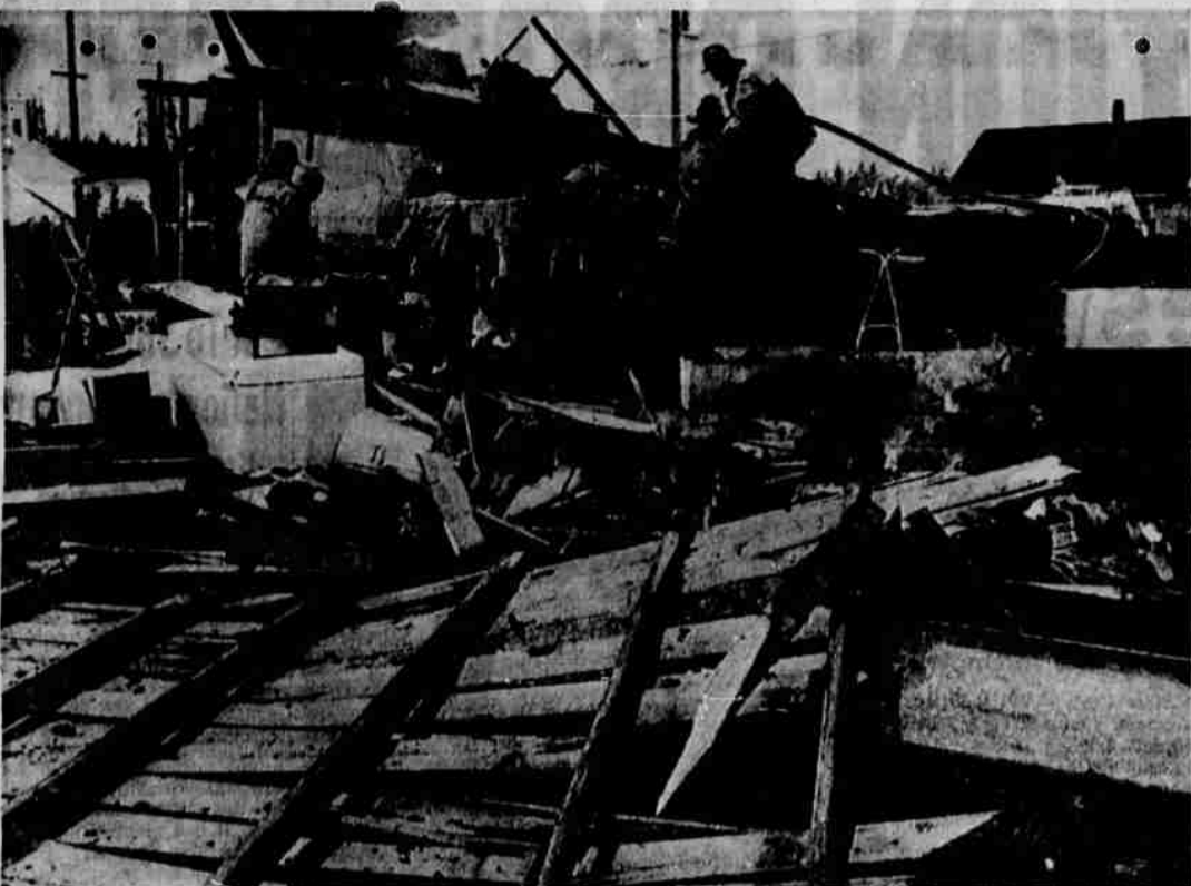
HOUSE DESTROYED —A natural gas explosion destroyed this home in northeast Portland. The Rev. Lyle O. Wilson, 30, pastor of the Sunrise Baptist church, was listed in satisfactory condition in a Portland hospital despite burns, cuts and bruises inflicted when he was pinned by a falling wall while working in his yard at the time of the blast.
