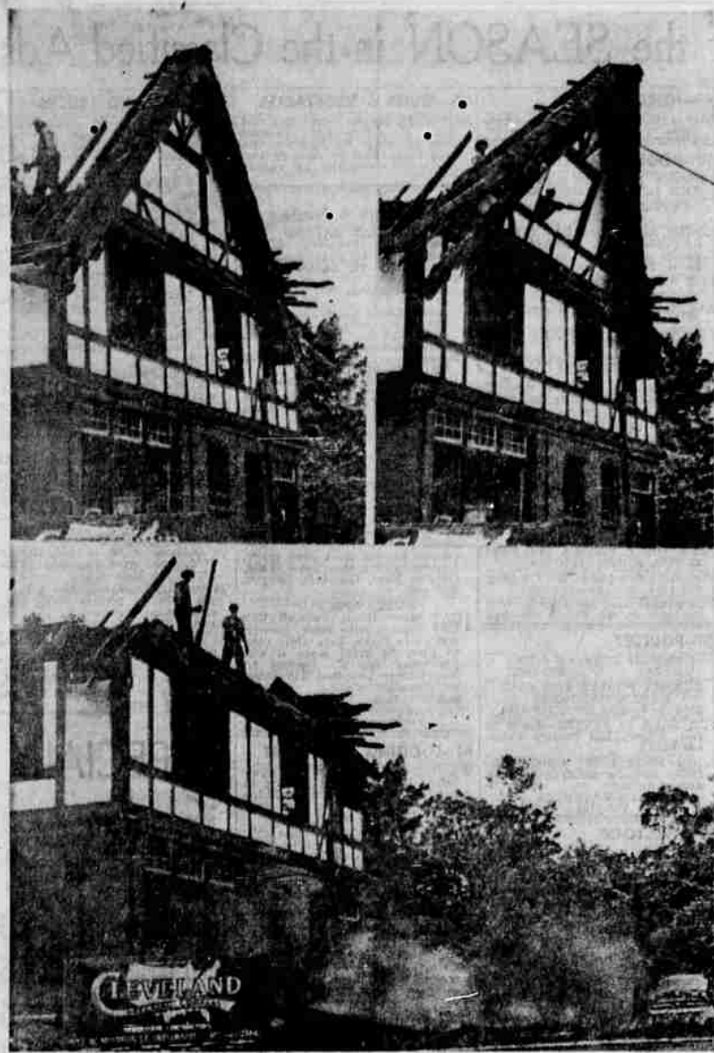
MANSION WRECKED - The old Indiana governor's mansion falls victim to the wreck-er as the land is cleared at Indianapolis for a parking lot. It was used by governors from 1919 to 1945. (UPI)
