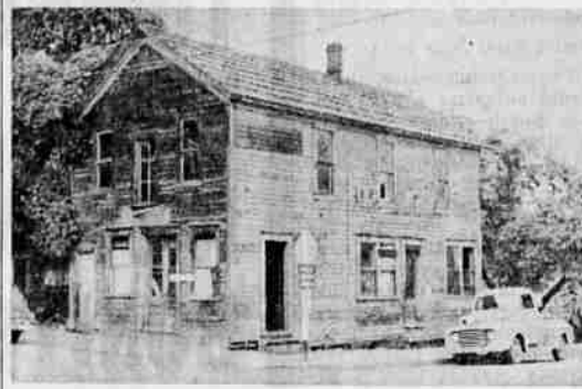
IN 1962—This was the Lyden House about three weeks ago just before it was torn down.
