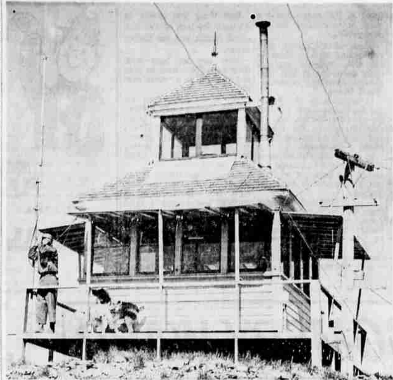
LOOKOUT HOUSE —This is the present lookout house. The fine is in the cupola, and the vertical rods Dutchman Peak lookout house. The fine are radio-telephone antennas.
