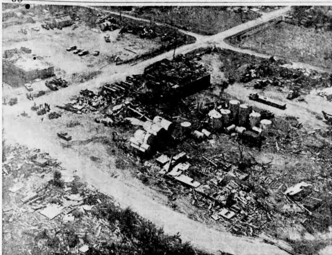
TORNADO BATTERS TOWN —A tornado cut through the west end of Mitchell, S. D., and sent more than two dozen people to hospitals but no one was killed. The district en-
