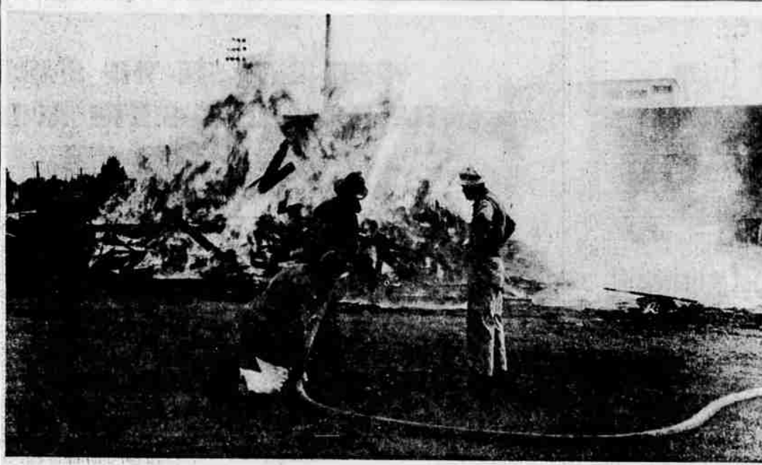
GRANDSTAND BURNED —The old wooden grandstand on the west side of the Medford school stadium has been torn down, and this morning firemen stood by while debris was burned. A new grandstand will be built in its place in time for use this fall. Funds for the new grandstand have been solicited from interested valley residents, eliminating use of tax money for it.
