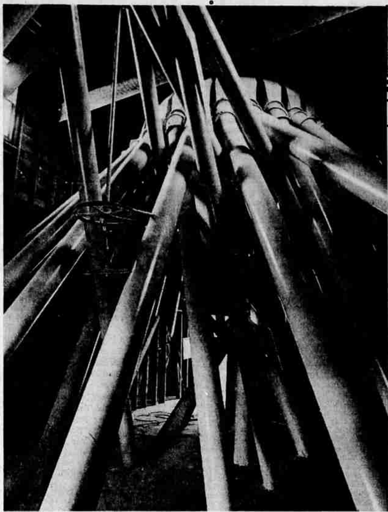
DISTRIBUTION SYSTEM — Some of the distribution pipe on the two top levels of the storage and feed manufacturing facility of the Grange Coop in Central Point is shown in this Anders Photo shop picture.
