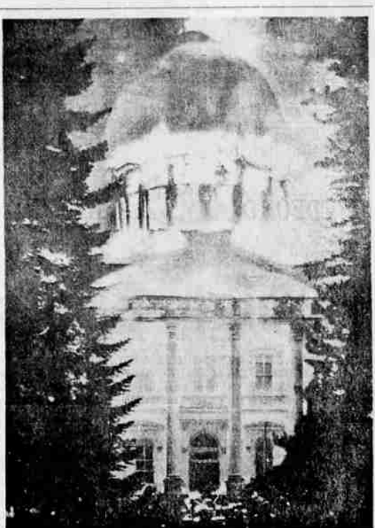
ANNIVERSARY OF FIRE —Today is the 27th anniversary of the fire which ruined the Oregon state capitol building in Salem on April 25, 1935. The photo above, from the Oregon State Archives, shows the building at the height of the fire. The story is on page 13 A. (UPI)
