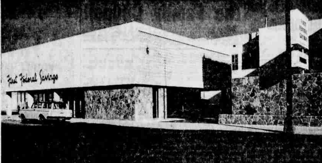
OPEN HOUSE — First Federal Savings and Loan Association's new building at the corner of Sixth and Grays sts. in Medford will be open for public inspection Saturday, April 28. The new structure was designed by Robert
