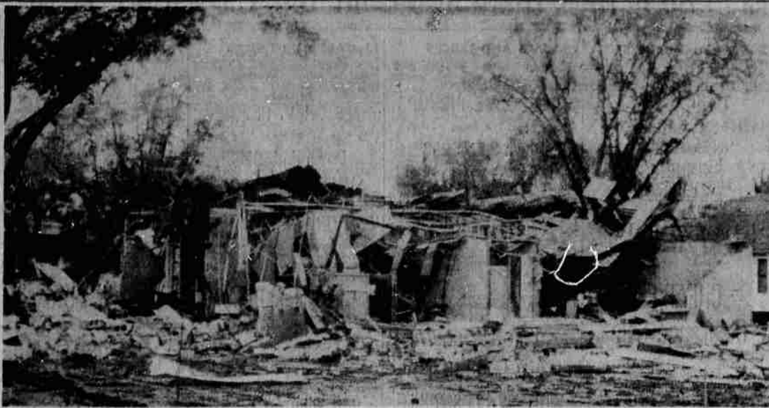
BANK DESTROYED - This general view shows the debris of a new bank building at Halstead, Kan., after an explosion Wednesday. The new building had been in use only since May 15. Although there were no deaths, eight
