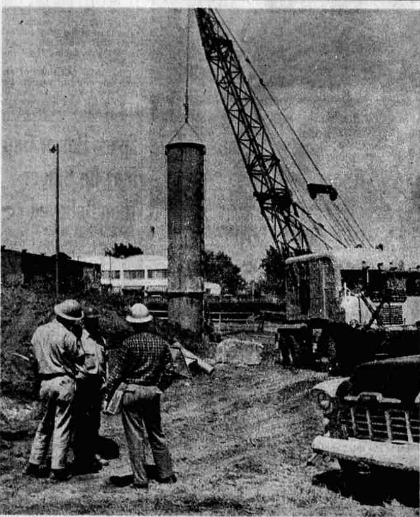
FREEWAY CONSTRUCTION —One of the huge supporting pillars for the freeway set in place yesterday at the east end of the 8th st. bridge. With the pillar in place it is possible to visualize how the freeway will change the appearance of this section of town.
