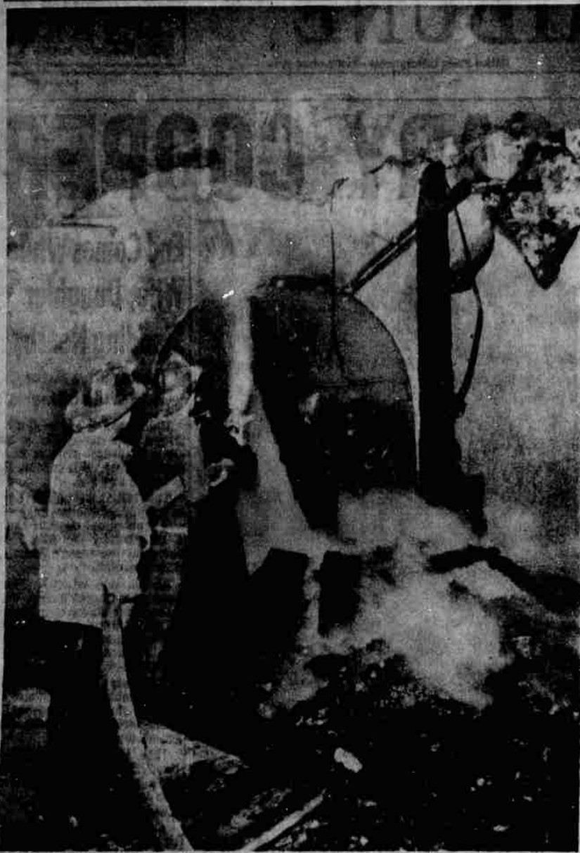
HOLLYWOOD HOMES DESTROYED — day and Saturday. At least 24 homes, a firemen spray water on a home that was completely burned by brush fire that swept through the Hollywood (Calif.) Hills Fri-
