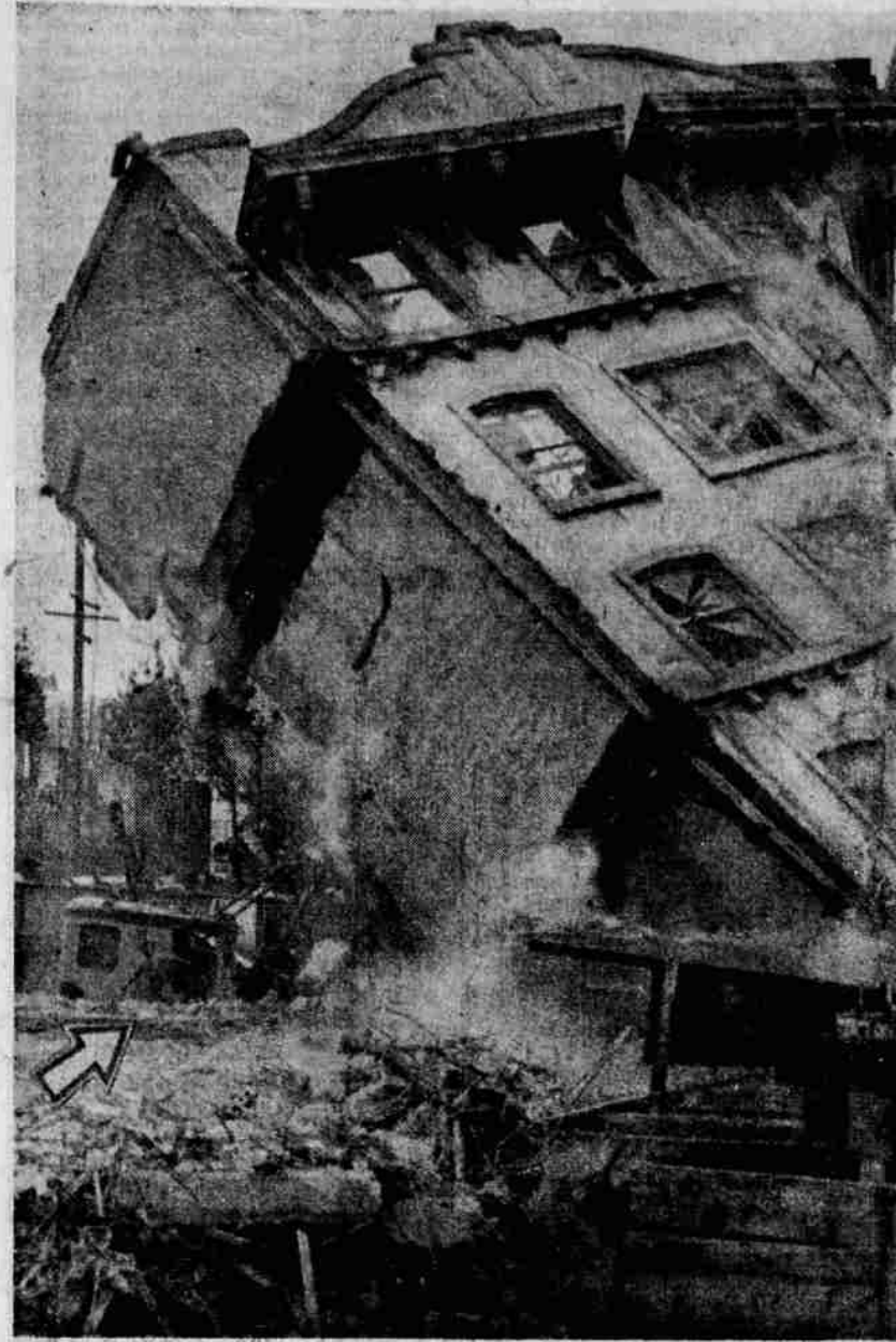
FALLING HOTEL—A surprised twist was taken by a hotel Saturday in urban renewal area near Portland as a bulldozer tugged at a cable to bring it down. Arrow points to the crane operator leaping from the cab to run for his life seconds before the building crashed at the foot of his crane. People watching the incident thought the crane operator was under the building and had to wait for dust to clear to discover he was safe. (UPI Telephoto)
