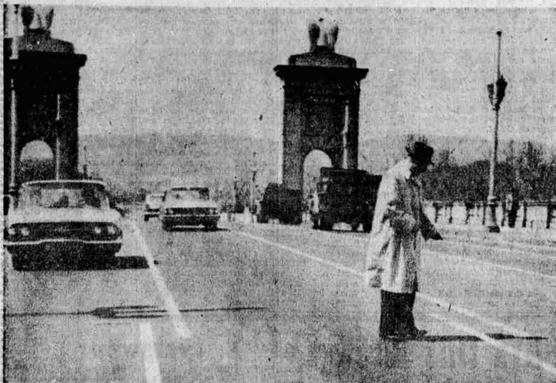
MISSED CONNECTION —Painters in Wilkes-Barre and Kingston borough, Pa., separated by this bridge, began painting traffic lines from their respective sides and scheduled a meeting in the middle. The meeting didn't come off
