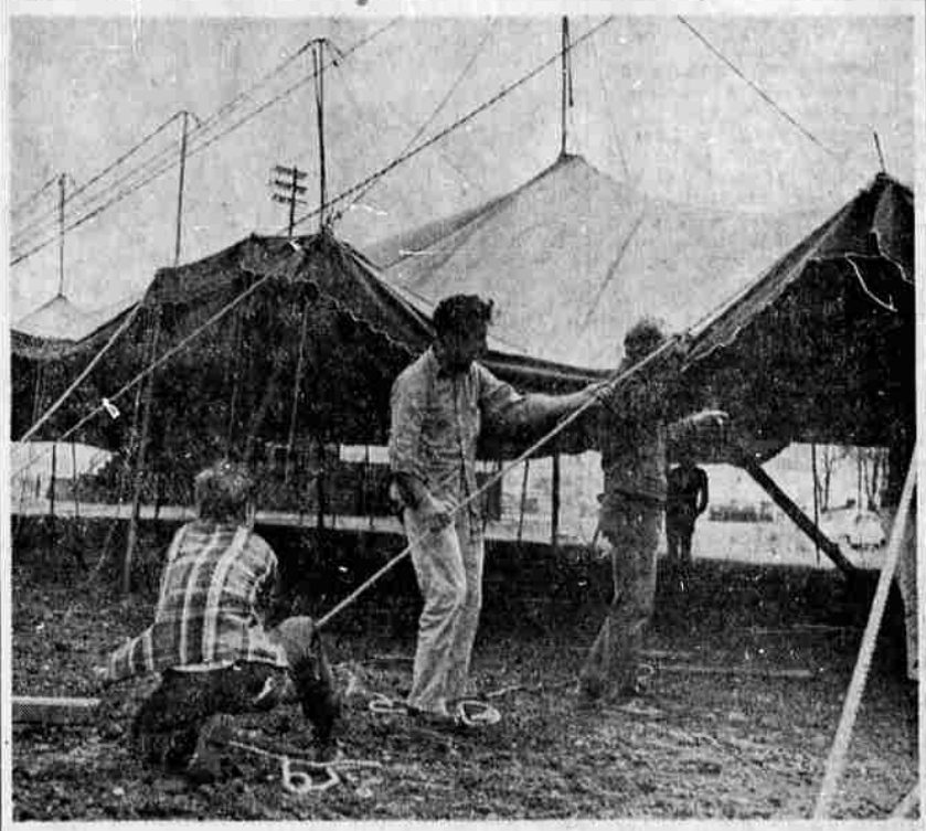
TENT ERECTED — Workmen above are shown as they put the poles under the giant tent that will contain exhibits of the Crater Lions club Sportsfair and Home and Garden show at the Medford armory grounds this week end. The event will have a larger number of exhibits than held in past years, according to Dick Hawkins, chairman of the show. Week end activities begin with a horse show and cutting contest in a specially-built arena southeast of the Medford armory at 8 p.m. Friday. Exhibits will include those of interest to sportsmen and home owners as well as youngsters.
