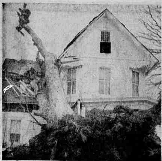
TORNADO DAMAGE —A tornado whipped through the central Illinois community of Winchester, causing an unestimated amount of damage. Here rescue workers "dismantle" a huge tree which impaled this house near the business district. The community of 1,800 persons was without power or telephone service for most of a day. (UPI Telephoto)
