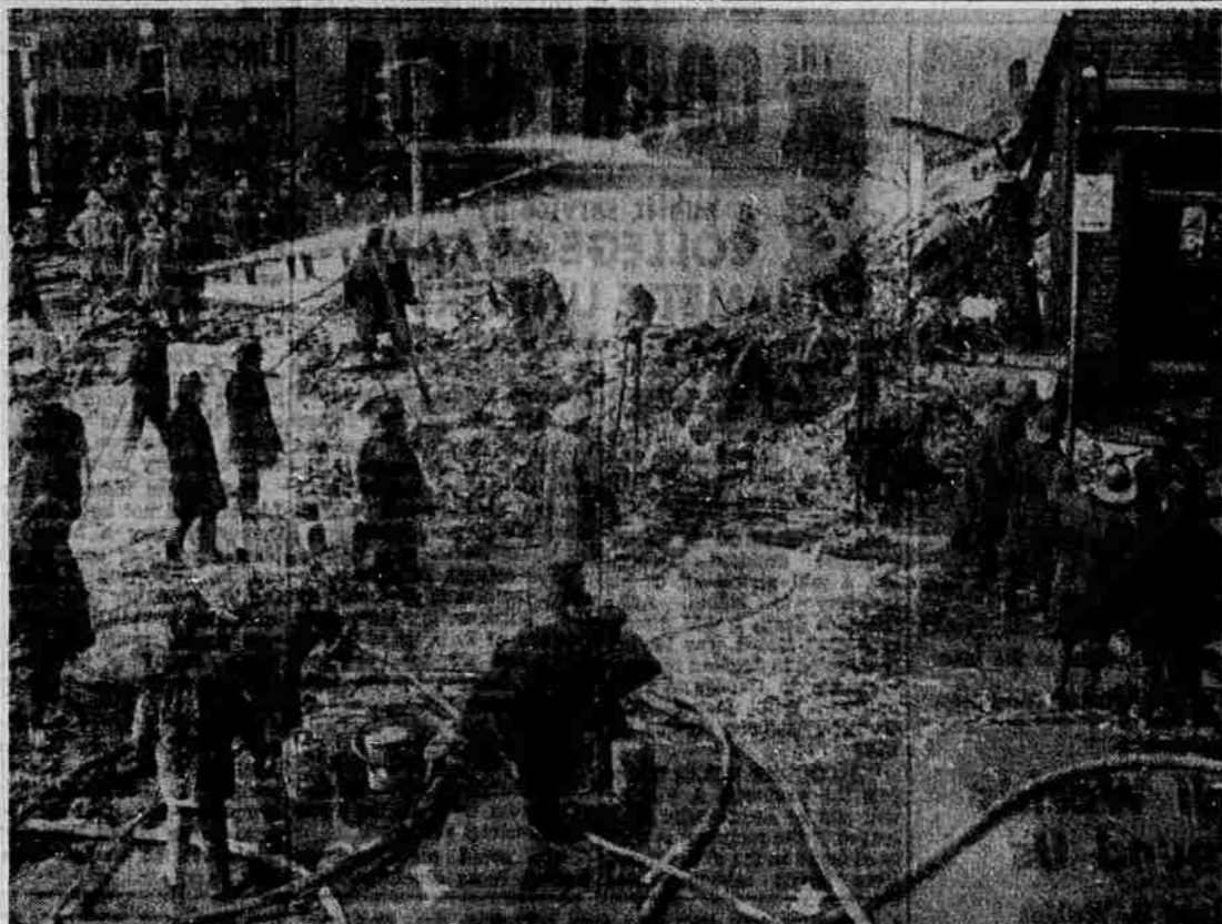
FIREMEN KILLED —A neighborhood gasoline station in Philadelphia exploded killing three firemen and injuring several others. More than 20 persons were injured in the blast. (UPI Telephoto)
