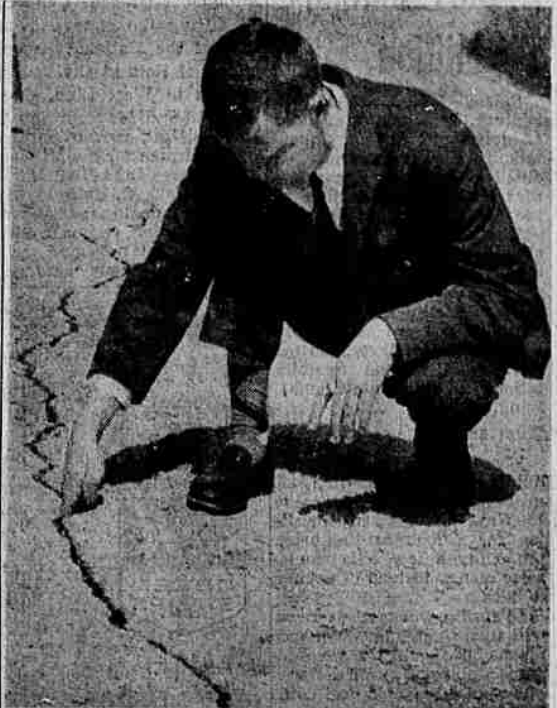
CRACK INVESTIGATED —San Francisco newspaper reporter George Murphy sticks his whole hand into a crack in the concrete in the highway west of Hollister, Calif. The crack was caused by an earthquake late Saturday. It was the worst quake in the Hollister area since the 1906 temblor. See picture on page 2.
