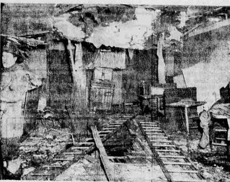
CHICAGO BLAST — This interior view shows blast damage after an explosion rocked a near north side night club in Chicago, Ill., late Friday killing one person and injuring at least 37 others. Fire officials said the blast was caused by a bomb. Five of the injured are in serious condition. —(UPI Telephoto)
