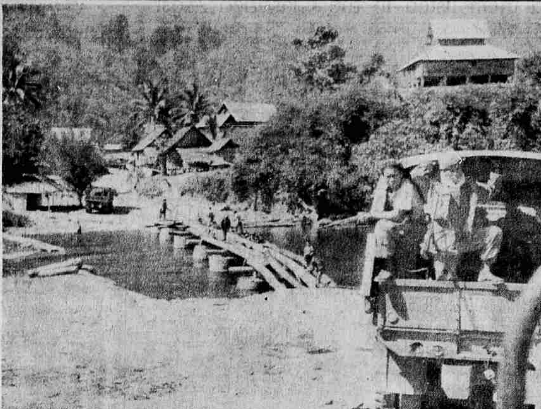
MAKESHIFT BRIDGE -Royal Laotian troops use logs to construct a makeshift bridge over the Nam Song river at Ban Pha Tang, Laos, recently after the former bridge was destroyed by Communist rebels. In the foreground, armed soldiers peer from truck as they await completion of the
