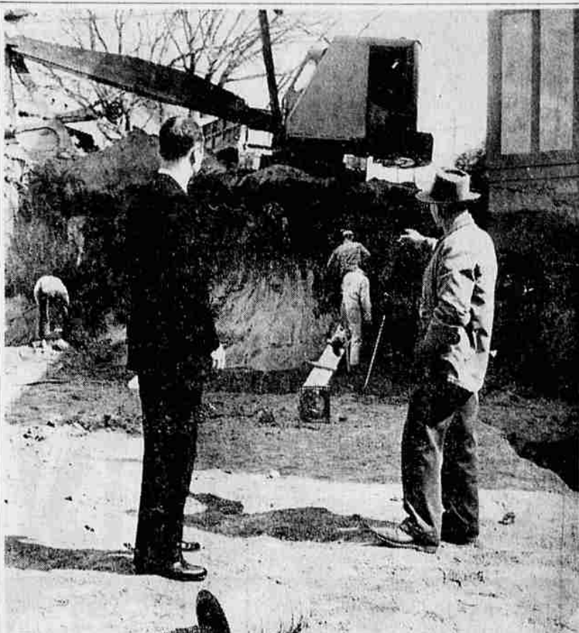
THEATER ADDITION —Excavation is progressing on the basement section of a new wing for Ashland's Shakespearean theater. The wing is part of a long range expansion program. The basement will house a costume workshop and will be used for additional rehearsal space. William Patton, wing for Ashland's Shakespearean theater, left, festival manager, and C. E. Corry, Lithia park superintendent, are shown checking progress.
