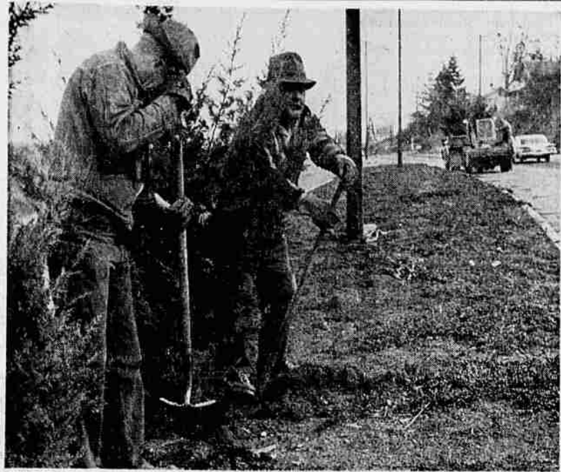
TREES REMOVED — A number of evergreens were removed from a traffic island between North Main and Glenn sts. on Highway 99 in Ashland Monday. R. L. Lammert, state highway department district superintendent, said the trees were removed at the request of Ashland residents, because the trees blocked the view of oncoming
