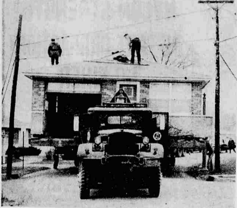
MOVING PROBLEMS — Making the day interesting for a moving crew at St. Louis, Mo., this five-room bungalow takes up most of the available space while being maneuvered down a street. The 70-ton house cleared the utility poles with inches to spare but the street lamp suffered damage. The house was being moved to another neighborhood. (UPI Telephoto)
