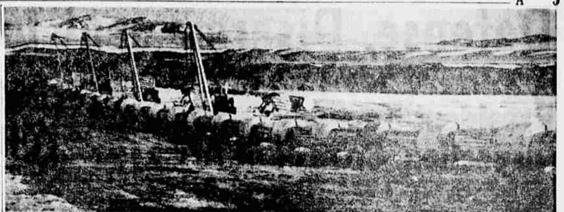
PIPE LINE LAID—Not sausage links but pipe for a river crossing on the 1,400-mile Alberta-California natural gas line is shown above in the eastern foothills of the Cana- dian Rockies near Calgary. The 36-inch-diameter steel pipe, fitted with concrete weights to overcome buoyancy and wooden slats to give protection against rocks, is ready to be "walked" by bulldozers into a trench at the bottom of the Oldman river which runs through the gully at cen- ter. The $30 million pipeline will bring Canadian gas to
