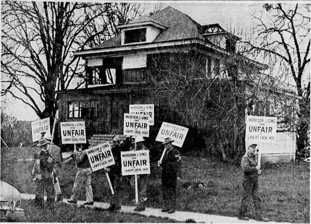
PICKETS — Members of the local Laborers union are shown as they picketed the construction site of the Alpine Village development in Medford yesterday afternoon. The picketing, still going on today, is a protest by the union against what they term "unfair labor practices" being employed by the demolition contractor. The building in the background is the old Osteopathic hospital, which is one of the structures being torn down to make room for the million-dollar development.
