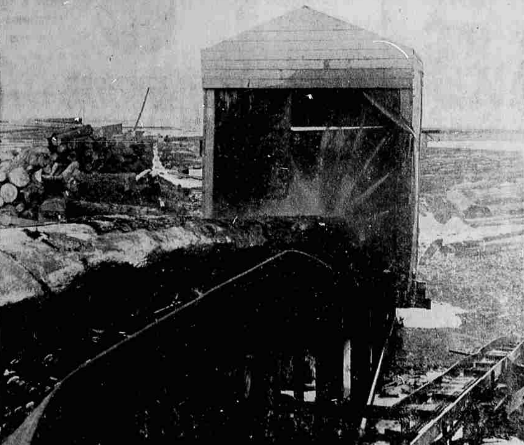
THROUGH SPRAY - A log moves through a series of sprays and along a moving belt into the Timber Products plant. The spray knocks off all mud and rocks which may
