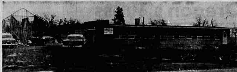
FIRST CHURCH OF GOD —Although construction is continuing on the new building for the First Church of God, 2000 Crater Lake Ave., the congregation has been holding services in the completed unit at right. The first unit, according to the Rev. W. E. Martin, pastor, includes six classrooms, a pastor's office and study and the fellowship hall. Completion of the second unit is scheduled for June 1.
