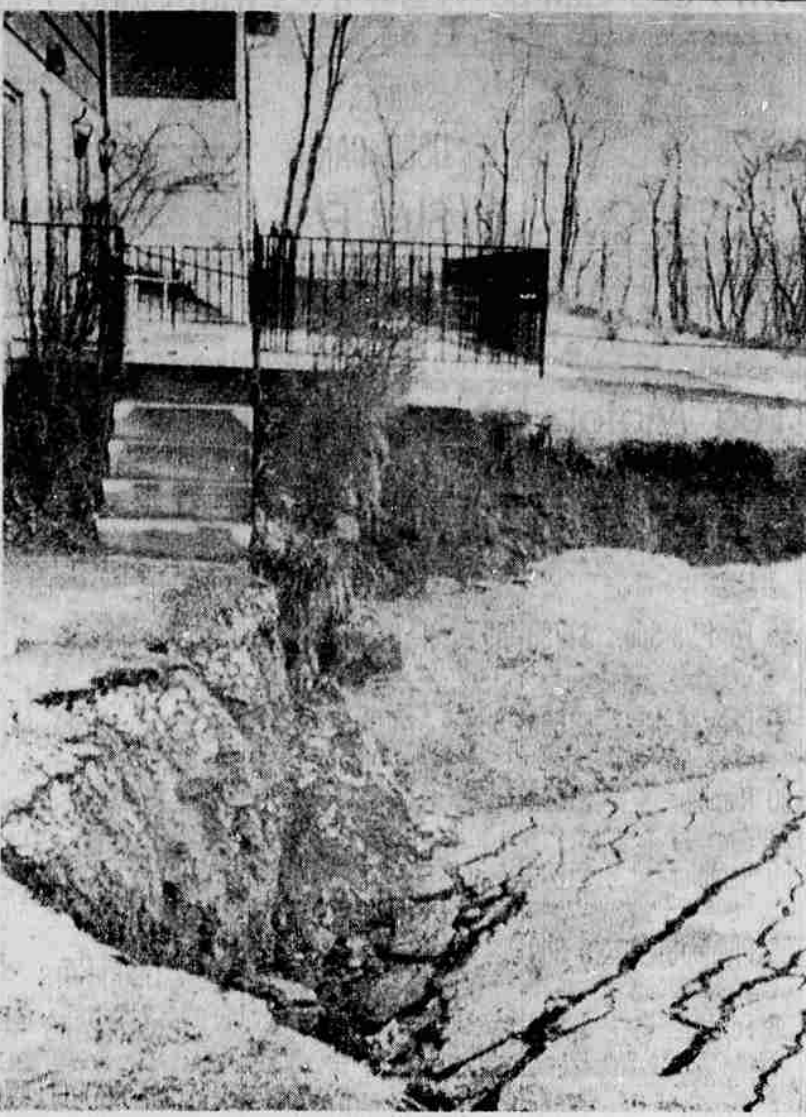
REALLY MEANS IT — When the Herman Schwartz family of Cynwyd, Pa., invites friends to "drop over some time," it could be quite a drop. Off the porch, it's 12 feet. A crack in the rock wall of a quarry opened fissures in the earth which have widened six inches daily. Earth has been sinking in the area about 12 inches daily. Homes have been evacuated and industries shut down, but nobody knows when the sinking will stop or how to stop it.
